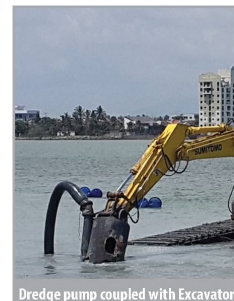
Dredge pump coupled with Excavator
